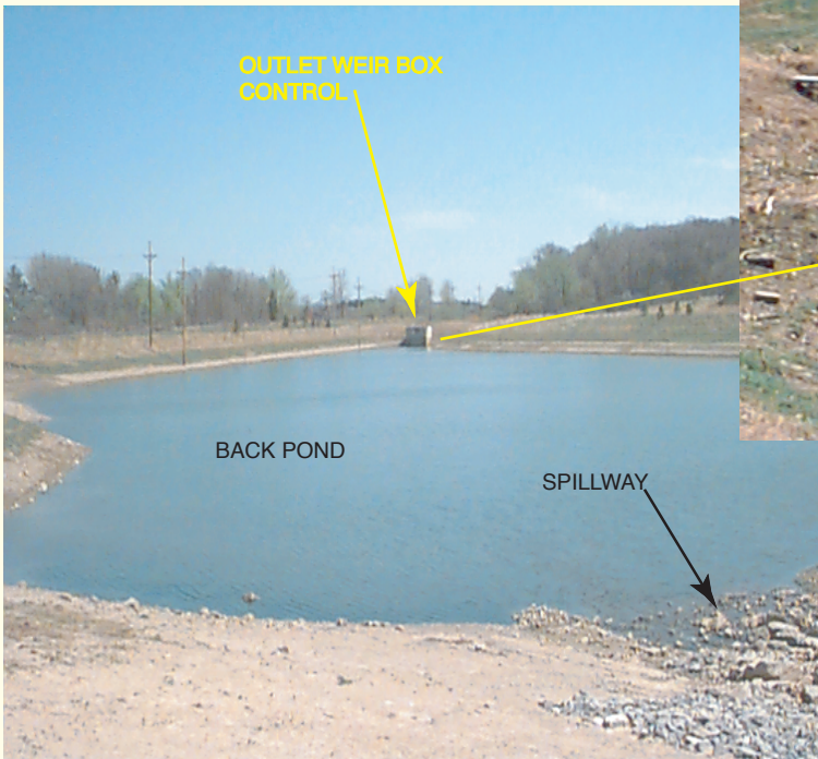
Figure 3. View of Jefferson Road detention basin in Town of Pittsford, N.Y.: A. View of back pond from spillway (also shown on front cover). B. Outlet weir box (also shown on back cover).
