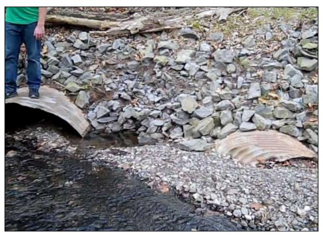
Figure 5. Upstream erosion of glacially laid gravels regular deposit at these twin culvert pipes on South Glen Road, Irondequoit, NY
